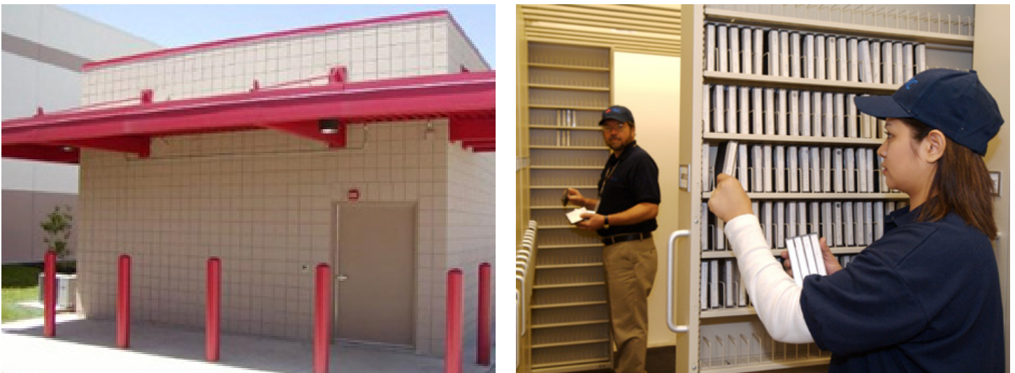
FIGURE 3. As an important lesson learned from Hurricane Katrina in 2005, NARA designed and built an Electronic Records Vault (ERV) for storing Federal agency essential records away from the most disaster prone areas of the country. The ERV is a secure, controlled access, environmentally controlled storage unit for Federal agencies' essential electronic records. Photos credit – NARA – Federal Records Centers Program
